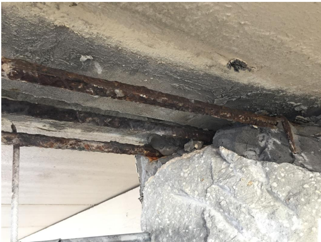
Picture 2: In-progress demolition of beam running in the North/South direction
