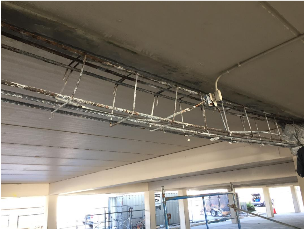
Picture 1: In-progress demolition of beam running in the North/South direction
