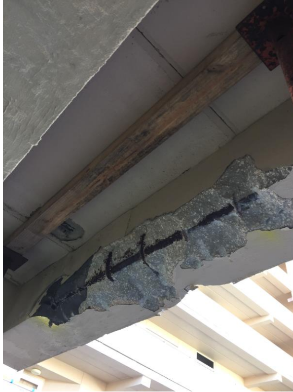
Picture 3: In-progress demolition of beam running in the East/West direction
