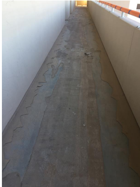
Picture 5: In-progress walkway stripping
